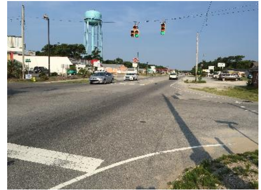
The intersection of 58 th Street and East Oak Island Drive does not provide adequate crossing facilities for bicyclists or pedestrians. Image Source: HCP, Inc.
