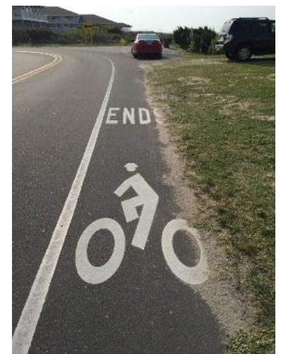
Debris, sand, and landscape material is encroaching upon cyclists traveling along the existing Beach Drive bicycle lane. Image Source: HCP, Inc.
